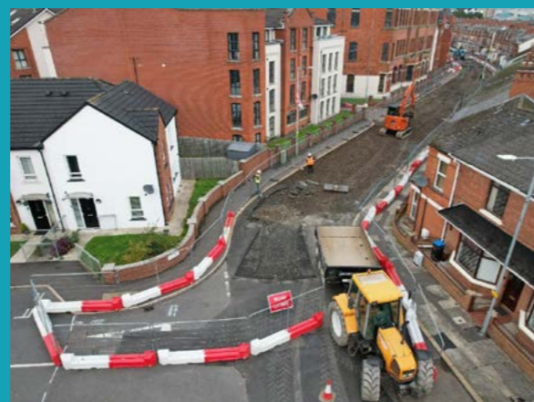
Ravenhill Avenue Flood Alleviation Project nearing completion.
