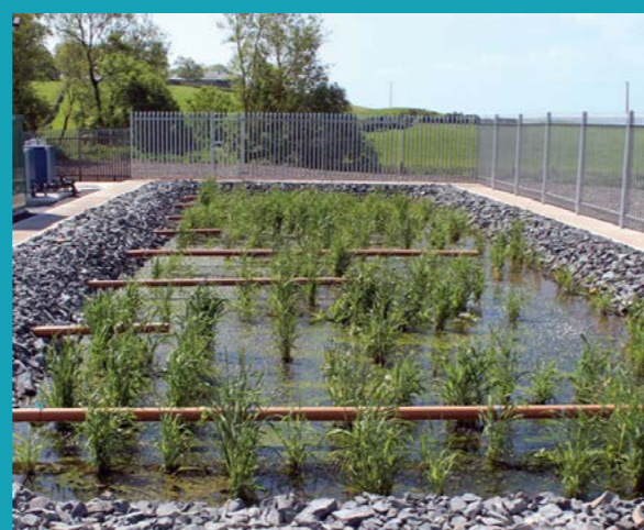
Aerated reed bed growth at Loughries wastewater treatment works, Newtownards, County Down.
