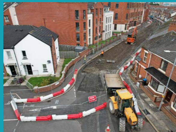
Ravenhill Avenue Flood Alleviation Project nearing completion.
