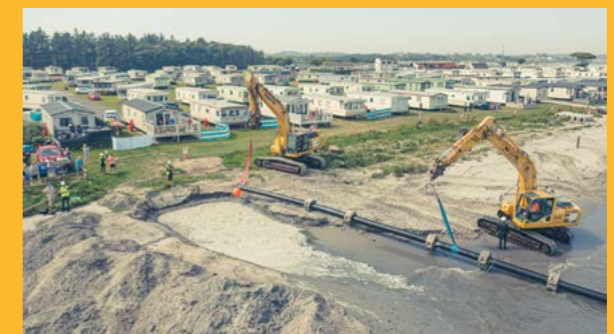
The long sea outfall during installation off the coast, adjacent to a caravan park at Ballyferris, County Down.
